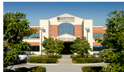
Northwest Medical Center – Willow Creek Women's Hospital, Johnson
